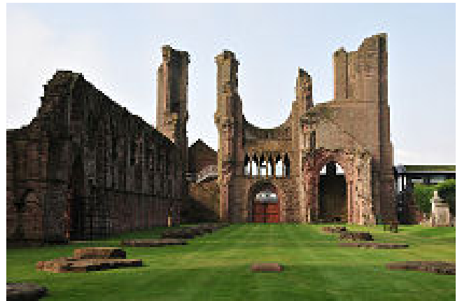
Nave Looking West
